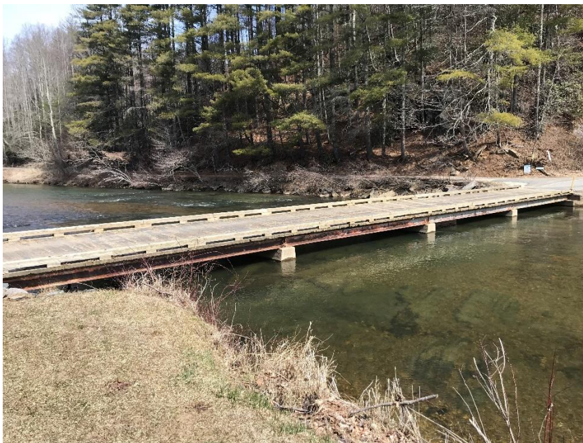
Photo 1. Bridge to be replaced across the South New Fork River, March 9, 2021.
